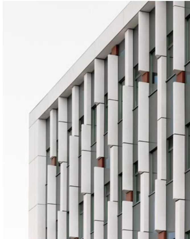
To secure non-visible fastening, an intelligent system with integrated fastening anchors was developed. Weather-proof pre-assembly in the factory guarantees a high standard of quality and rapid assembly on-site. The elements are simply hung into place and finely-adjusted into position.
